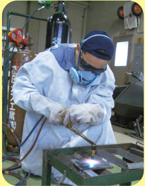
Gas cutting & welding
